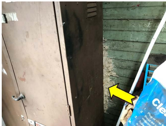
Photo 3. Interior, ground level, maintenance shed, east wall – non asbestos-containing vermiculite.
